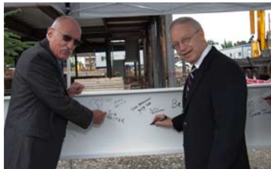
Ted Lewis (left), vice-chair of the Enumclaw Regional Hospital Board of Directors, and Dennis Popp, president of the hospital, sign the final steel beam before it is raised into place during the topping-out ceremony Aug. 11.
